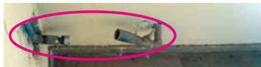
Figure 2. The water pipes had no connection
