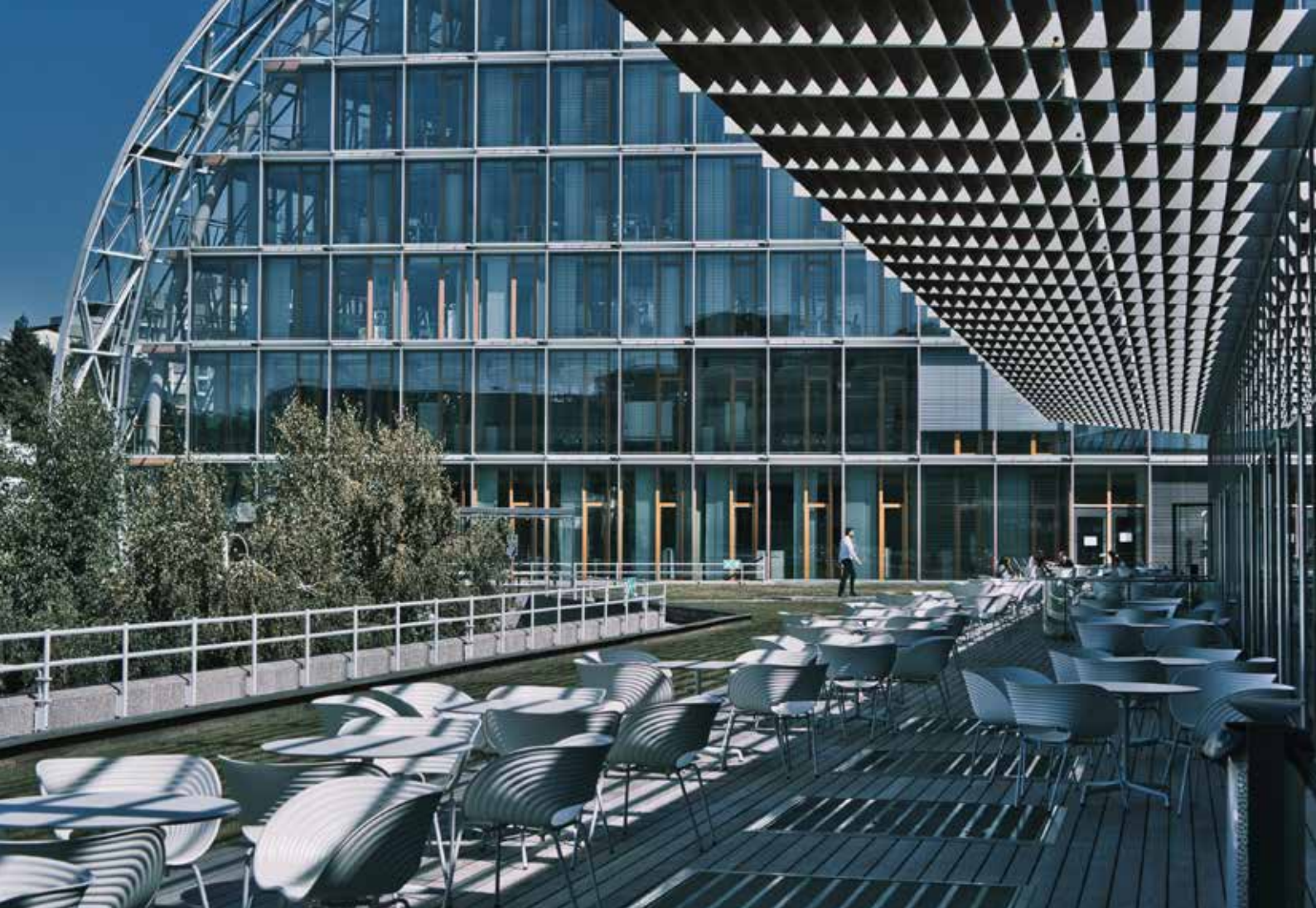
EIB EKI building. Photo taken by Marcel Serra, EIB employee
