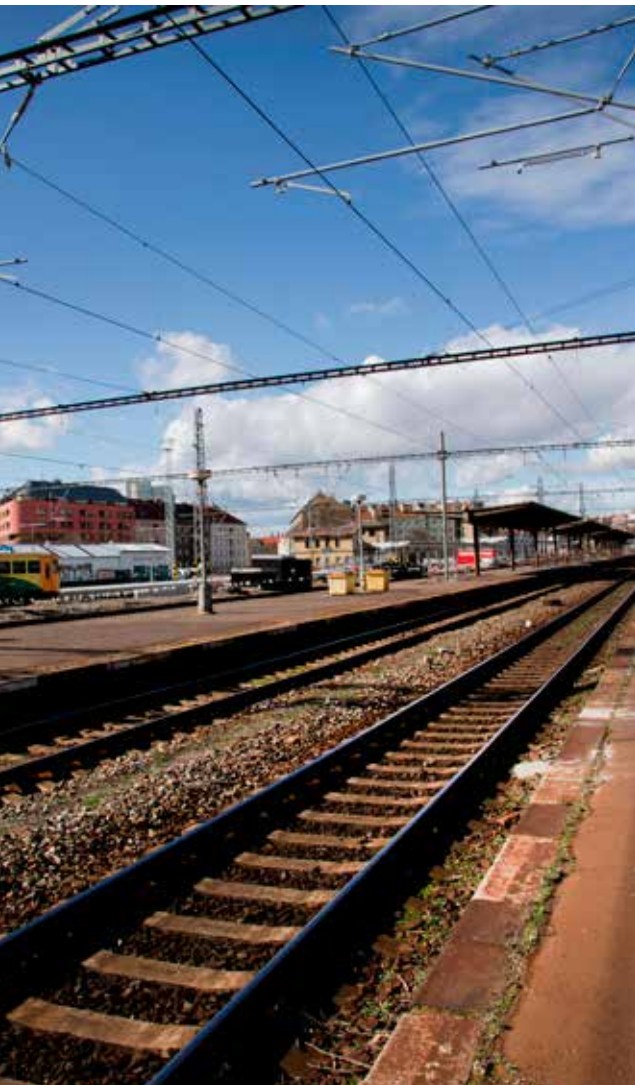
Prague railway infrastructure
