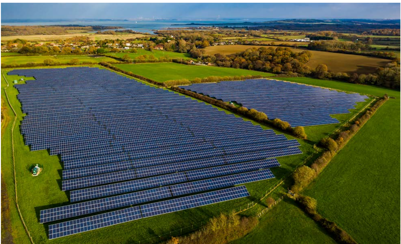
NTR solar plant in Ireland.
